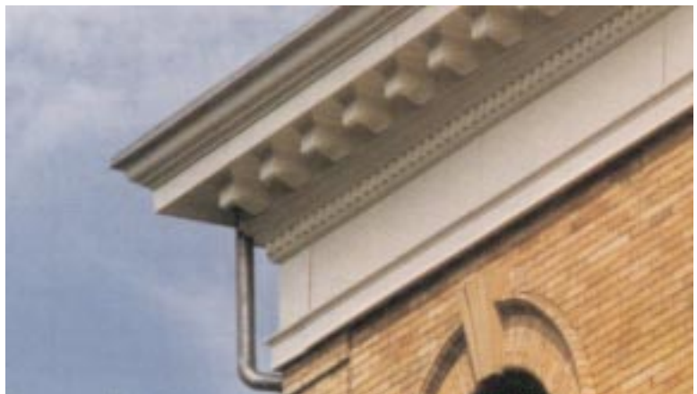
Example of cornice.
